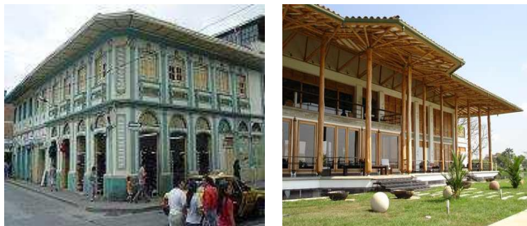
Figure 3: Bahareque style and modern Guadua bamboo house in Colombia (Simon Velez)
