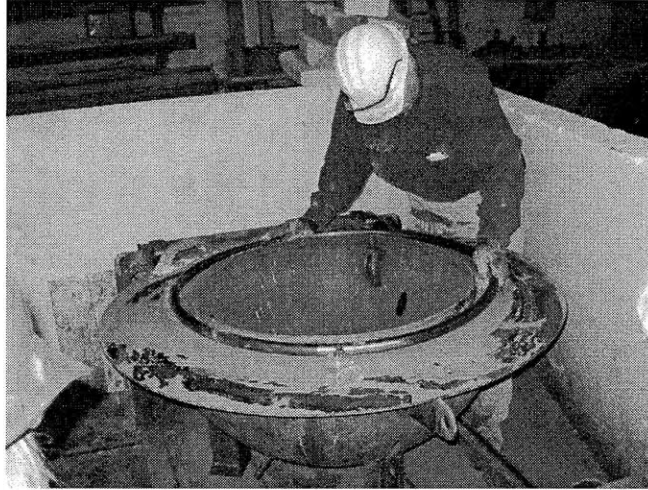
Figure 51: The studded steel ring being pressed into the concrete. The plastic wrap used in attempts to seal the backer rod can be seen on the stud in the foreground. This plastic wrap caused several problems during assembly.
