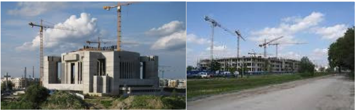
Temple (left) and Robyg (right) construction
