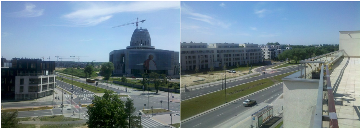
Temple & Office Park construction (left) & Rzeczospolita Avenue (right) - June 2011
