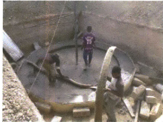
Figure 44: The forms are removed the next day
