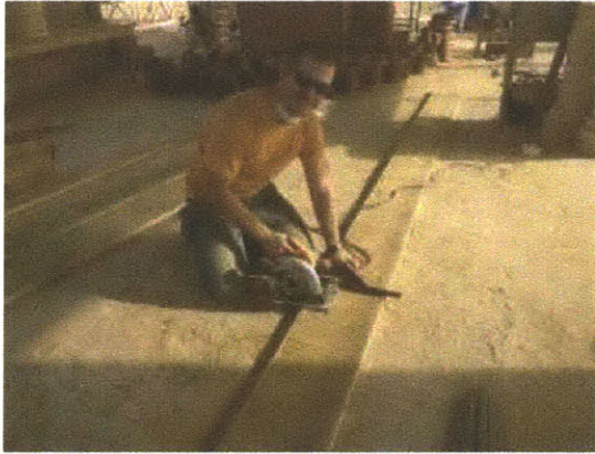
Figure 27: Mitch Westwood kerfs planks of wood for the formwork
