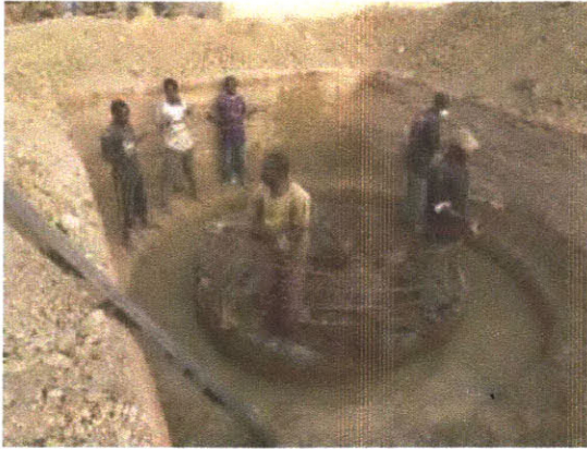
Figure 24: Rebar reinforcement lifted down into excavated area for the footing
