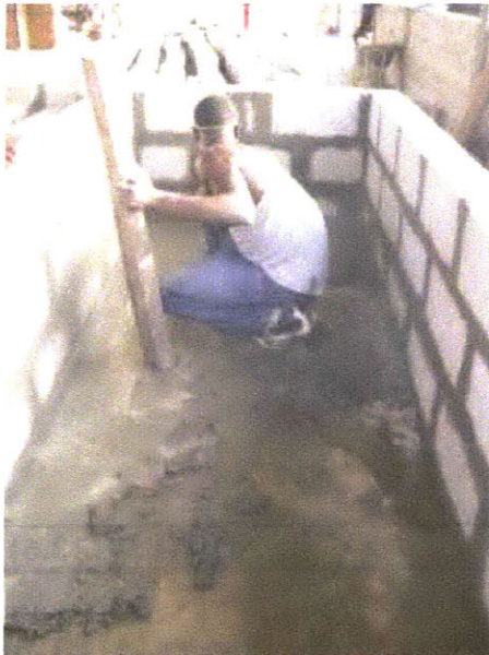
Figure 53: The mason slopes the floor of the tank towards the drain
