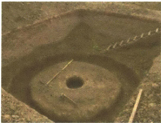
Figure 16: Footing and center hole dug and ready for 2-inch base layer center pole hole.
