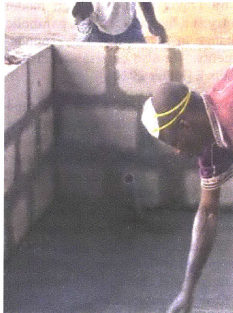
Figure 57: Outlet Detail – Grey drainage pipe (cap off) is also removable so that sludge from very bottom of tank can be cleaned out.
