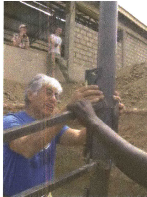
Figure 36: Securing and positioning pole exactly at tank center using a level and 4 cables
