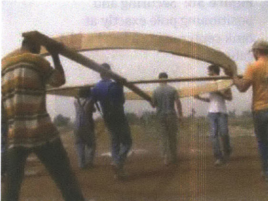
Figure 33: Carrying the inner form
