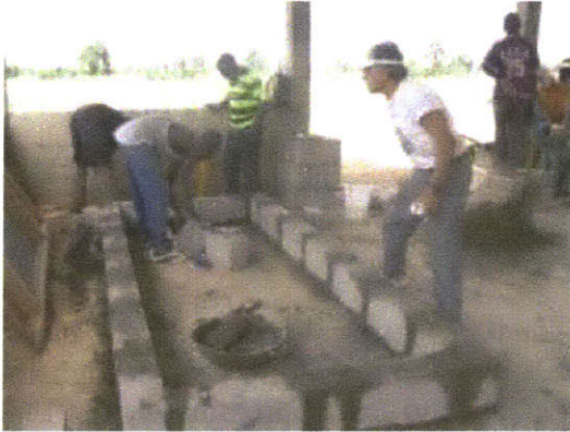
Figure 51: The mason lays the first row of bricks
