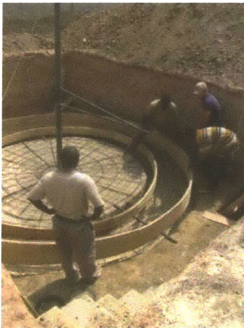
Figure 37: Using rotating arm on the center pole to ensure accurate placement of the inner form. Cutting a hole in the outer form for the placement of a 4 inch PVC outlet and drainage pipe
