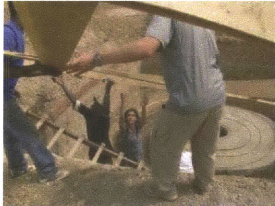
Figure 34: Lowering the inner form
