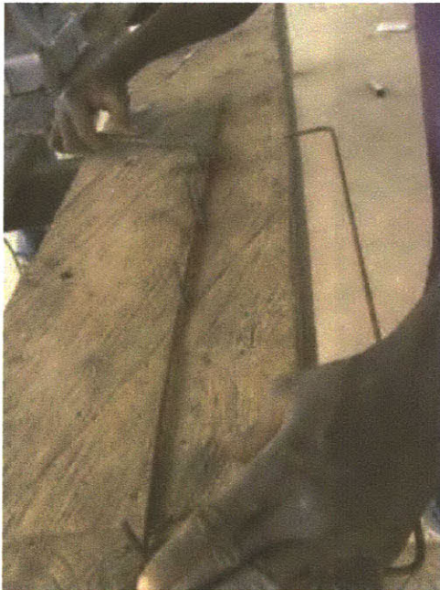
Figure 22: Close up of the jig used by the steel bender to bend rebar rod
