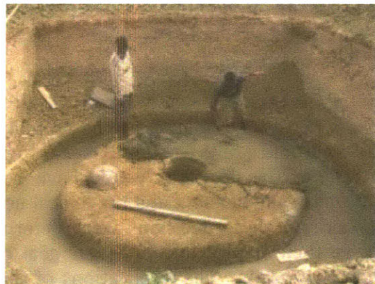
Figure 17: The mason applies a 2-inch base layer (1:3 cement to sand ratio) to the bottom of the footing, tank base
