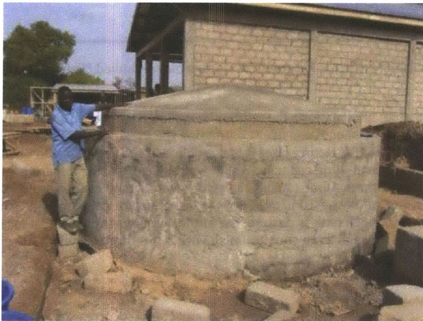
Figure 48: Post-January work: Tank walls are plastered with stucco
