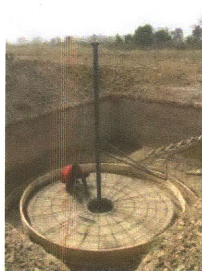
Figure 38: Roof support pole raised and centered. The steel bender continues work on rebar reinforcement
