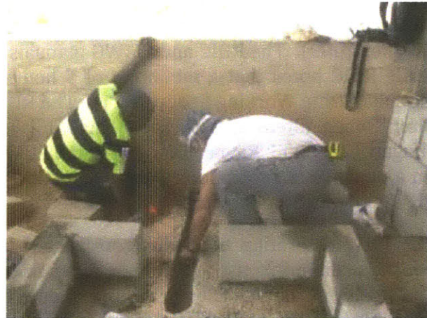
Figure 52: Manny Hernandez measures trench for the outlet pipe
