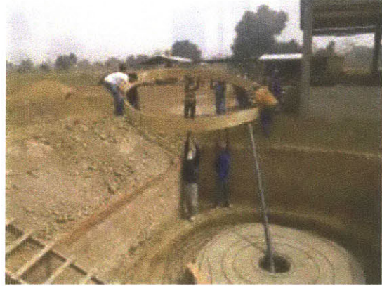
Figure 32: Lowering the outer form over the center-pole and around the rebar reinforcement
