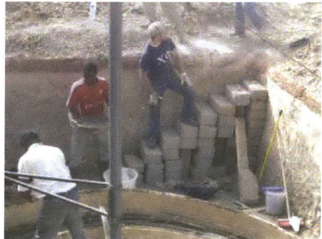
Figure 42: Foundation pouring happens one head-pan at a time. Westwood stands on the stairs ready to pass down another head-pan full of cement to Sadat, who passes to Mr. Kuma, to pour into the foundation
