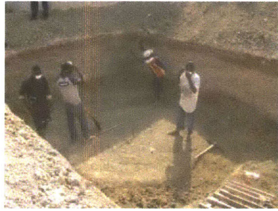
Figure 15: Using pic-axes to break up the ground and dig the tank footing
