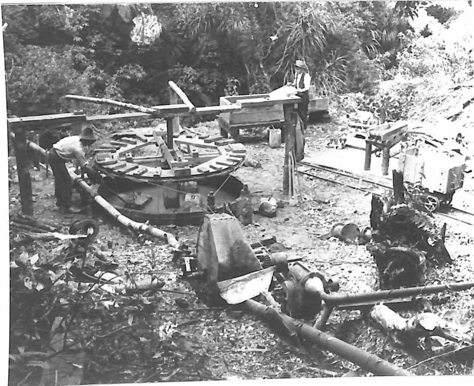
Figure 20: Malcolm Hardy and an assistant grinding ore, 1930s [two photos], David Calder Hardy Collection; used with permission.
