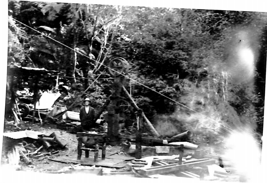
Figure 26: 'Side view showing pelton and belt drive. Smithy to left'.
