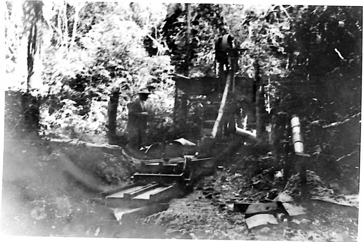
Figure 25: View showing plate & riffles. Water line passes down hill at back – 75ft fall.
