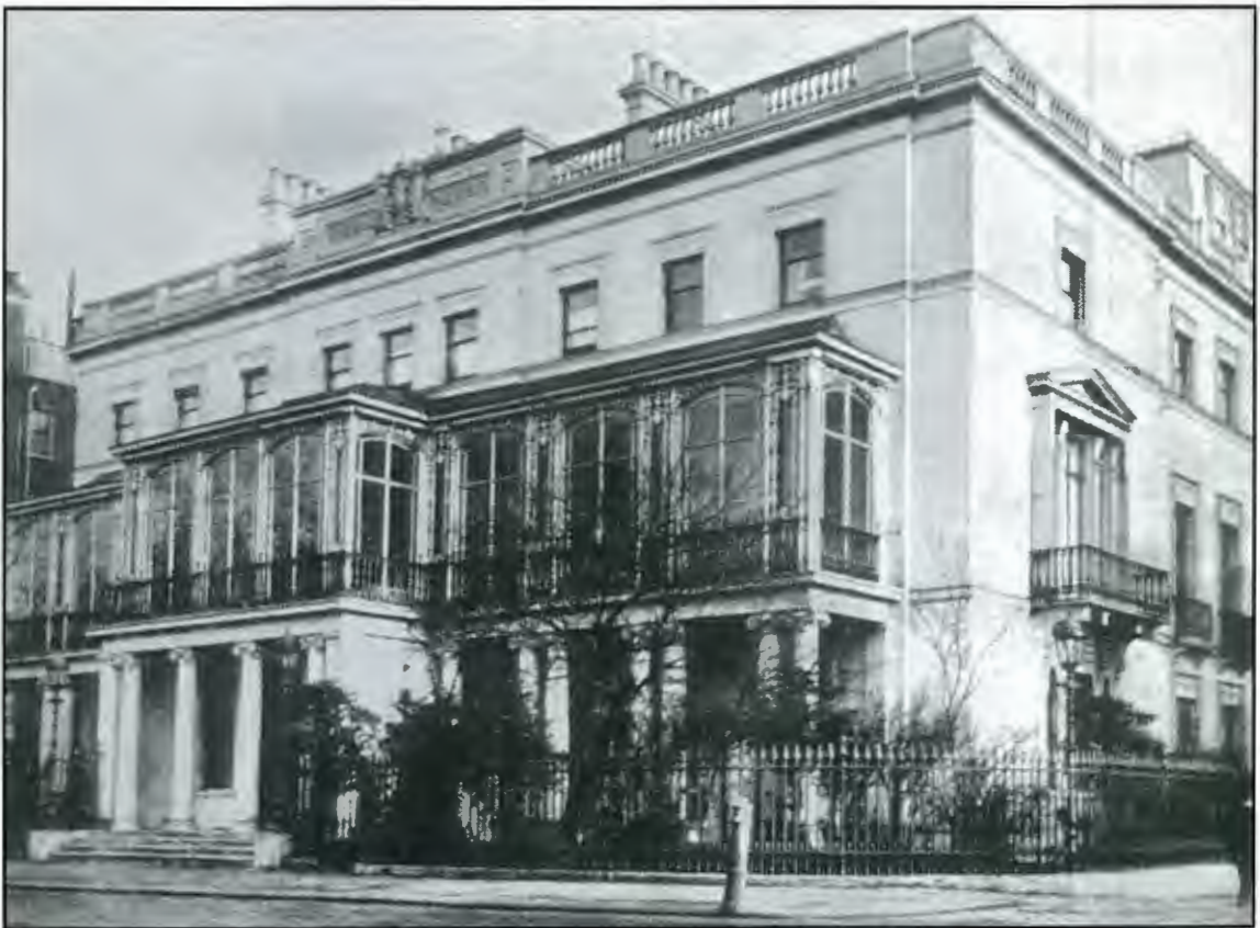
Figure 5.4 Dudley House, Park Lane, London
