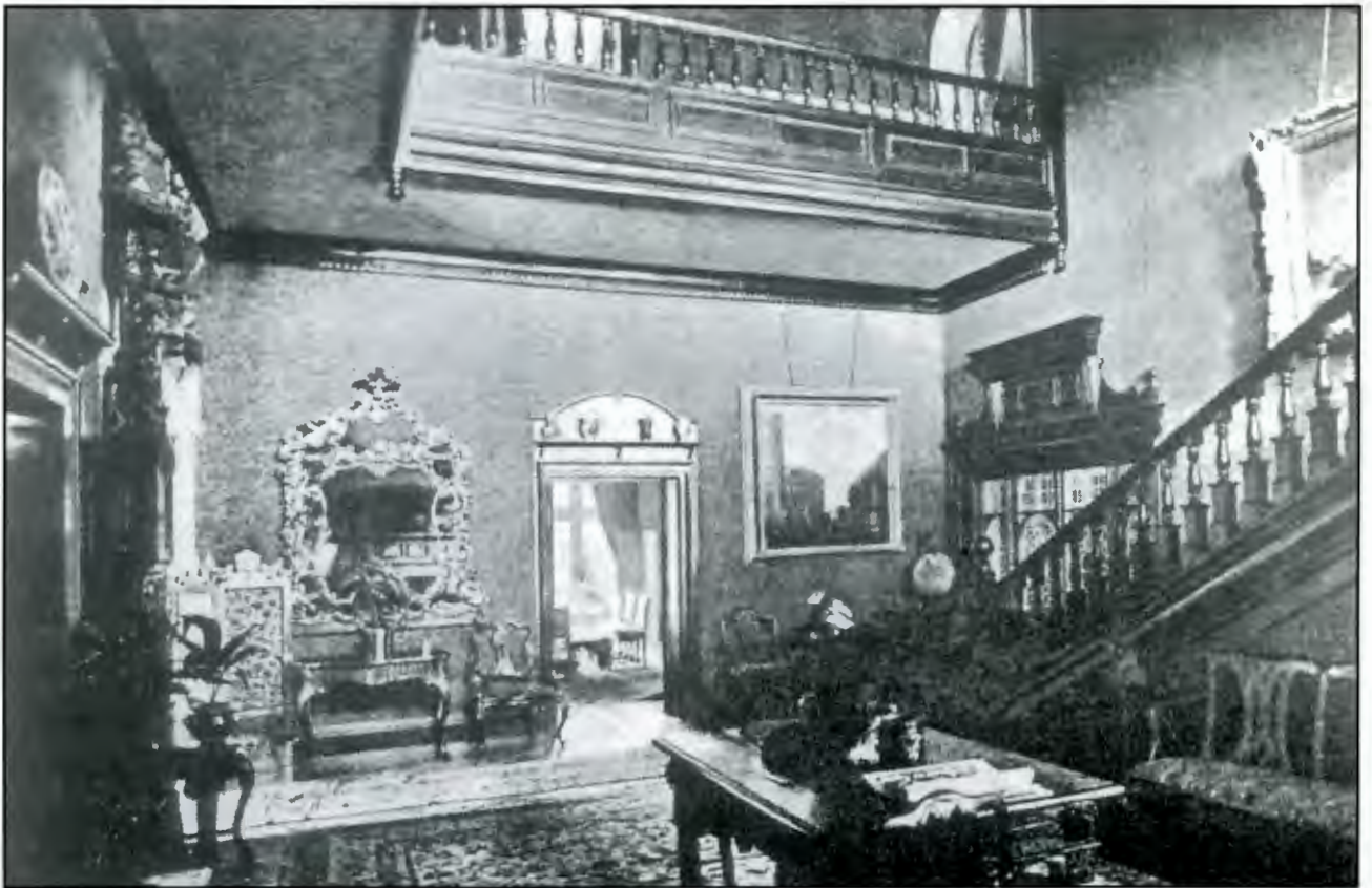
Figure 3.4 Interior of Hohenheim, Johannesburg
