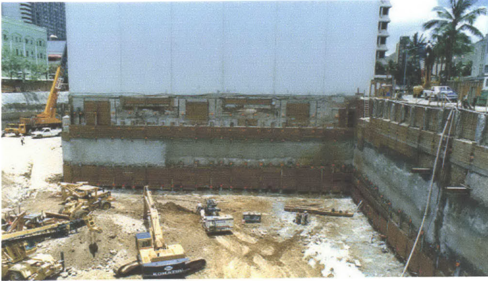
Figure 18 General View of Excavation Works, Honolulu [15]
