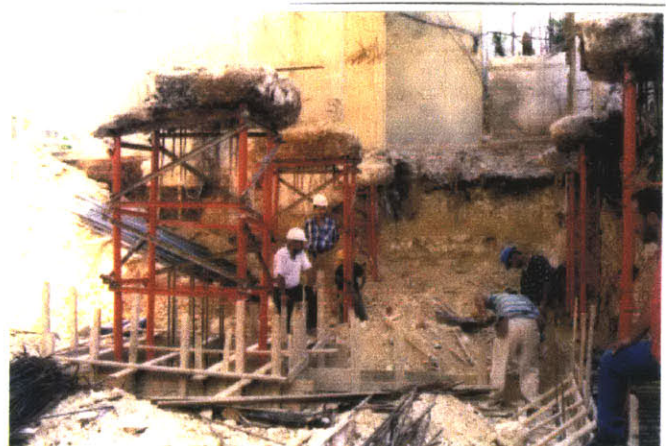
Figure 2 Underpinning Works [14]
