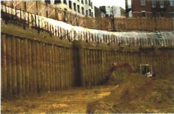
Figure 3 Shoring Structure [14]
