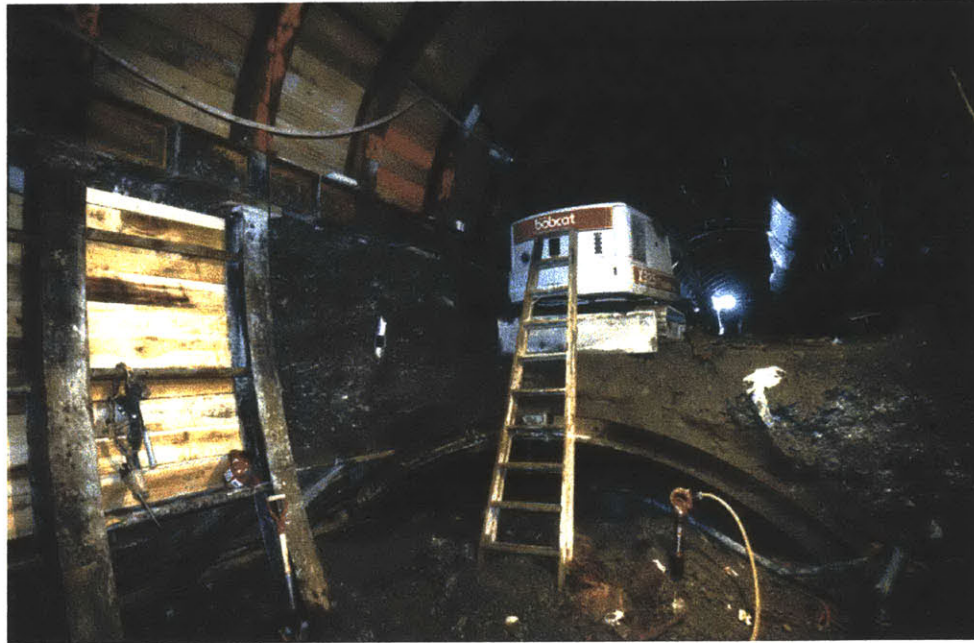
Figure 27 Inside drift tunnels under the Red Line subway at South Station [12]
