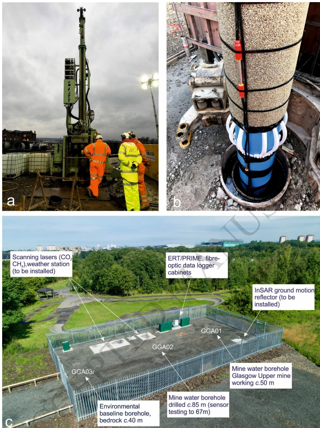
Figure 5 Images of (a) Drilling of the cored borehole GGC01 in 2018 (b) Installation of uPVC casing screen to mine water borehole with pre-glued gravel pack, electrical resistivity sensor cable (red sensors) and fibre optic cable. Photos a,b BGS©UKRI 2020 (c) research compound Site 1 at July 2020, background photo courtesy BAM Nuttall .
