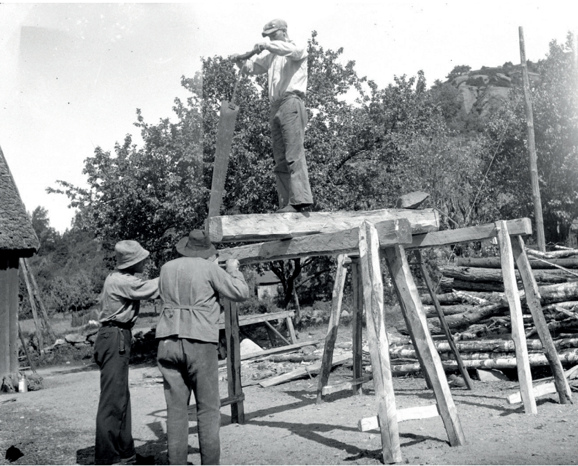
Fig. 8. The crane-saw is a large saw managed by two or more people to cleave logs into boards by hand. The noun crane has been interpreted as referring to the figure and movement of the large bird of that name: the saw's handle resembles the bird's long inclined neck, and the movements of the person managing the saw are like a crane's dance in spring. Photo by Albert Sandklef. Hallands kulturhistoriska museum.
