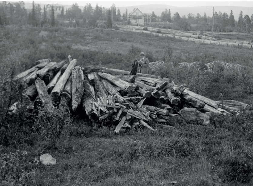
Fig 7. 1933, Olle Homman at the Nordic Museum taking notes and making drawings of the logs from the old chapel in Gråträsk, Norrbotten. In the background the new chapel is under construction in the traditional log timber technique. Photo by John Granlund, the Nordic Museums archive.
