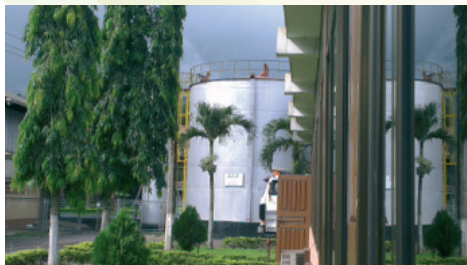
Figure 3: Agro-processing facility for palm oil
