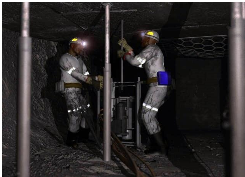
Figure 2.8C: Installation of a roof bolt in the hanging wall.
