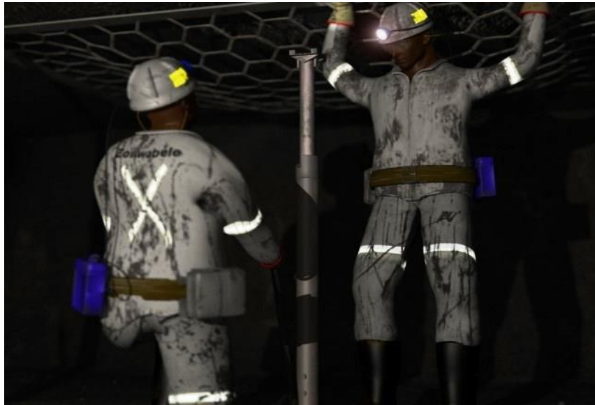
Figure 2.8B: Workers installing the safety net.
