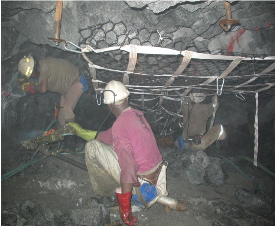
Figure 7.7: Rock netting installed at Impala No. 10 shaft.
