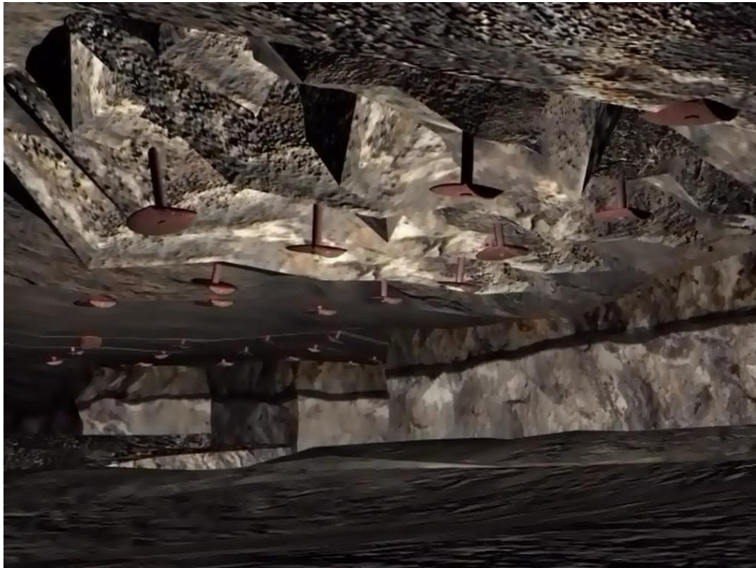
Figure 7.18: Blocky ground in the hanging near the stope face area.
