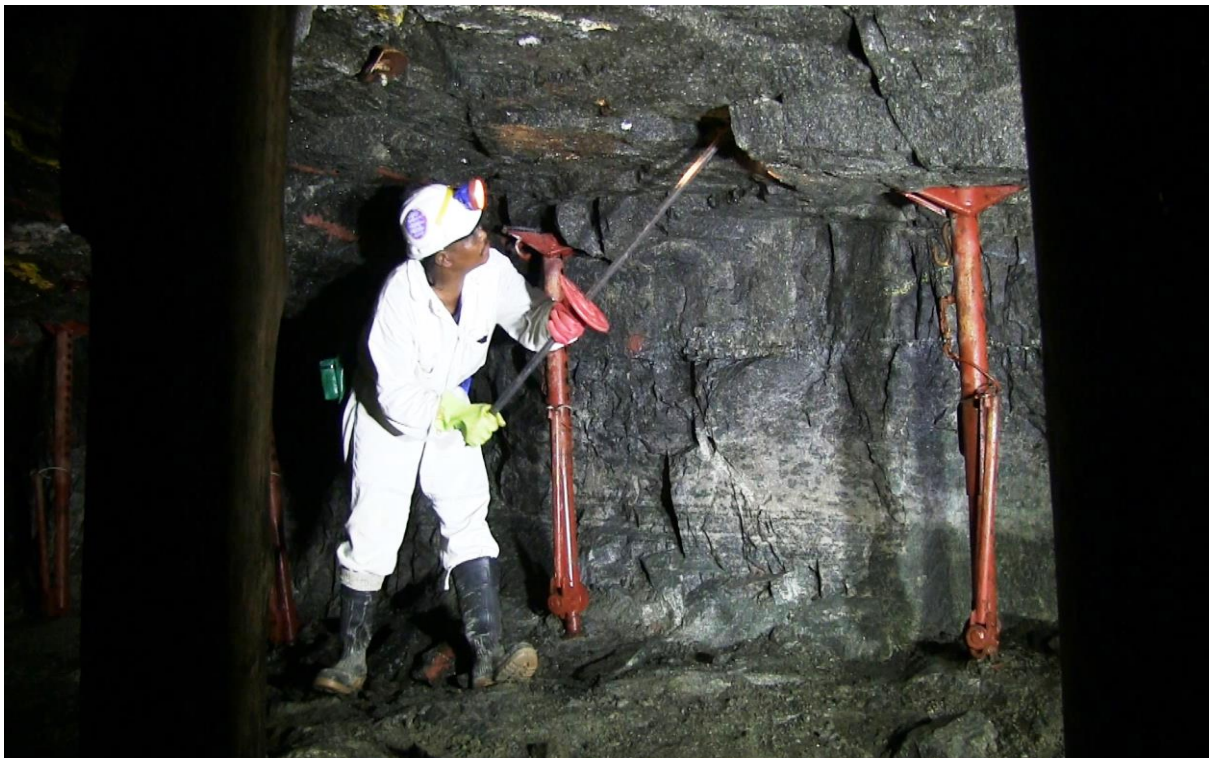
Figure 6.5: Worker using pinch bar to dislodge loose rocks.
