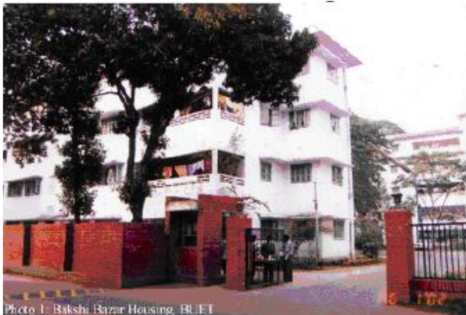
Figure-1.4: Housing at Buet Campus. (source: Hafiz, 2004)
