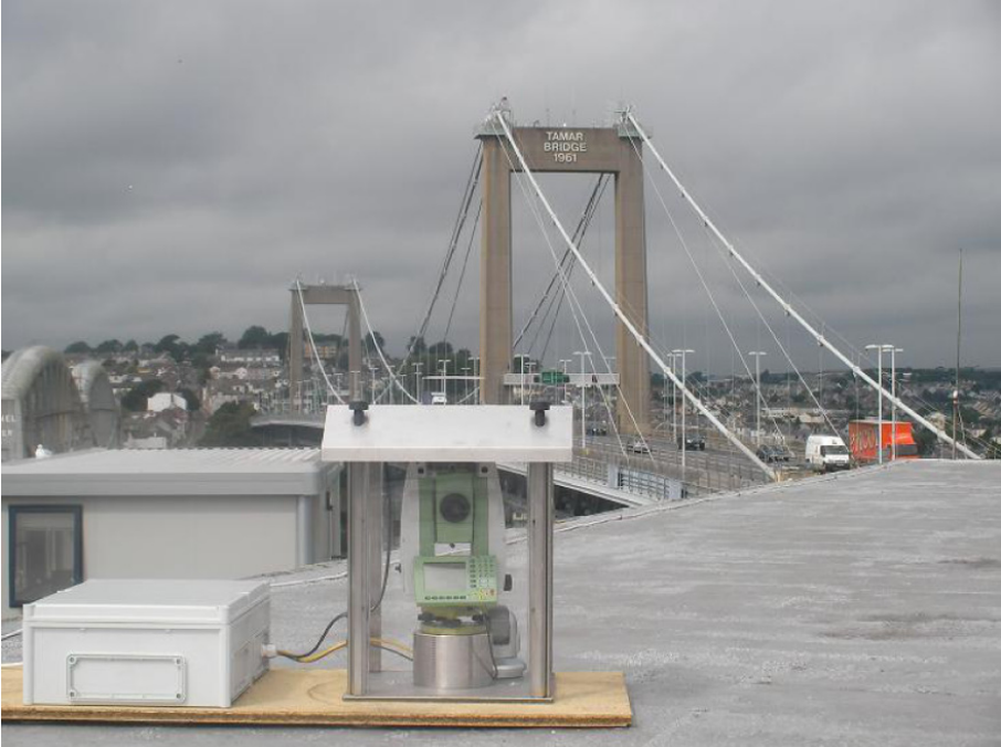
Figure 3: RTS installed on the roof of Tamar Bridge Office
