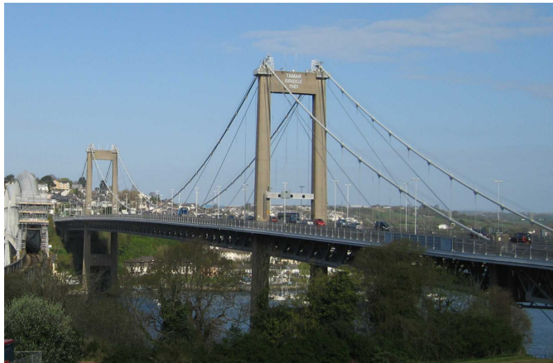
Figure 1: Tamar suspension bridge
