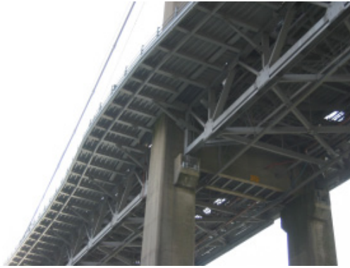
Figure 2: Cantilever lanes added in the upgrade
