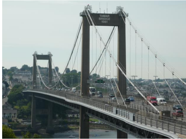
Figure 3. The Tamar Suspension Bridge
