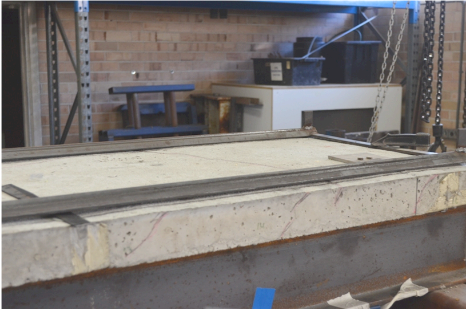
Figure 22 - Observed additional cracks in the second loading scenario
