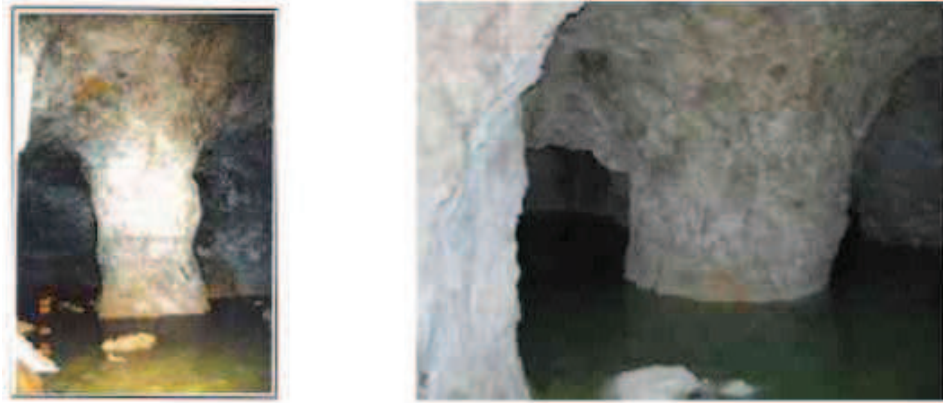
Figure 5.12: Views of a pillar in the Rocquevaire abandoned quarry (Bouches-du-Rhône, France) with two different water flooding level (left in 1996 and right in 2010, by courtesy of Watelet JM, INERIS).
