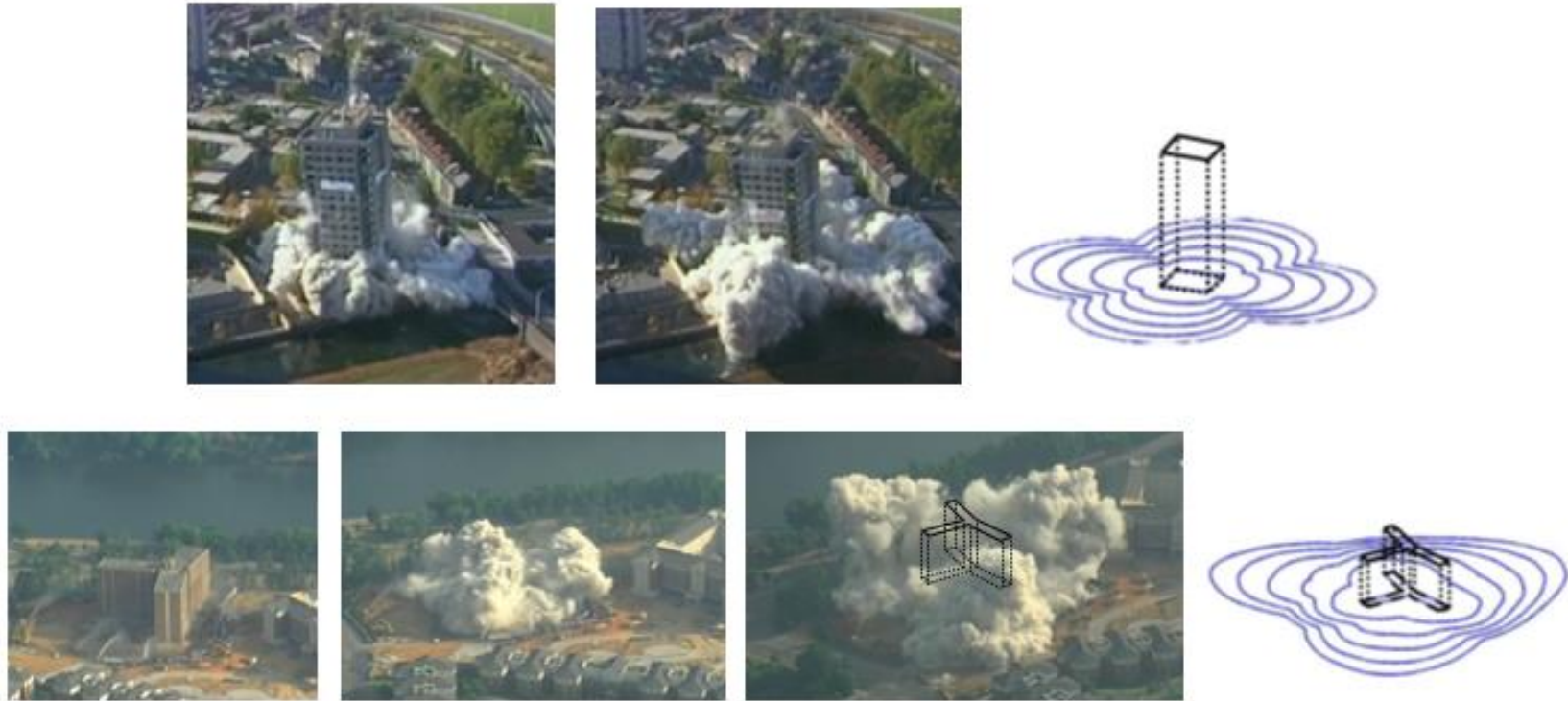
Figure 3-1. Field observations of a non-circular gravity current. Aerial views of (top) a building of square cross-section and (bottom) a T-shaped building being demolished. The structure of the debris cloud is highly dependent on the building's shape. Observe that material very close to the center of the building moves farther out than material located at the building's extremities. The dynamics of the cloud is reasonably well captured by our proposed model, where the front location of the cloud is marked at equal instants of time as blue lines.
