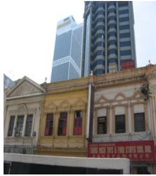
Figure 2. Lack of Harmony in the Colours of the Building Facades (Amir, 2007)
