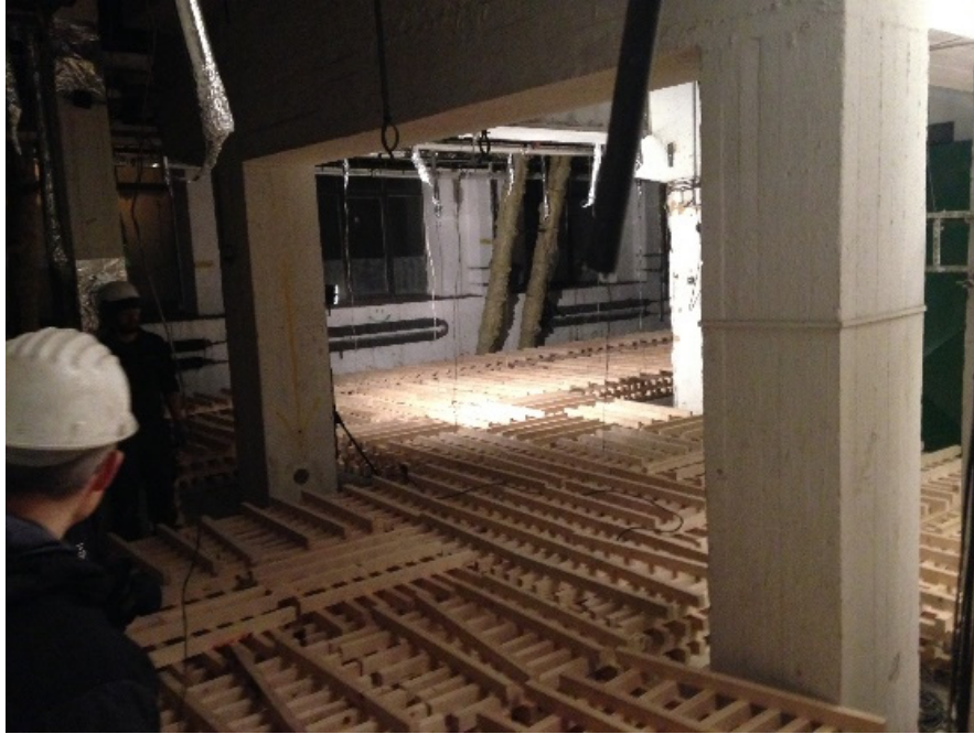
Figure 2.8. View inside of the Tisová travelling fire experimental compartment (photo provided by Rush D., Tisova Fire Test-2015, report forthcoming).
