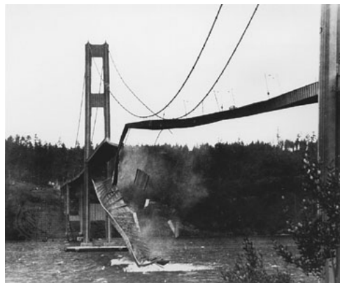
Figure 2.3: Tacoma Narrows bridge during wind-induced vibration. The bridge opened on July 1, 1940, and collapsed on November 7, 1940. (Farquharson photo, Historical Photography Collection, University of Washington Libraries.)
