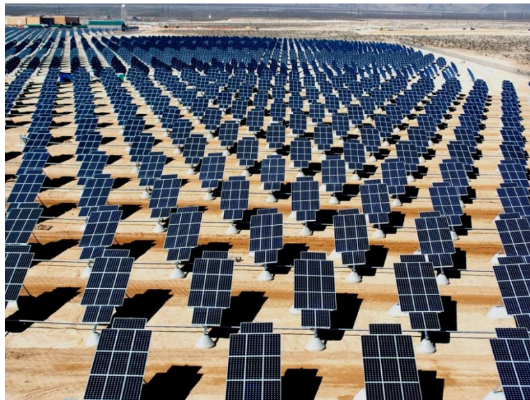
Figure 2.2: Solar PV arrays [2].
