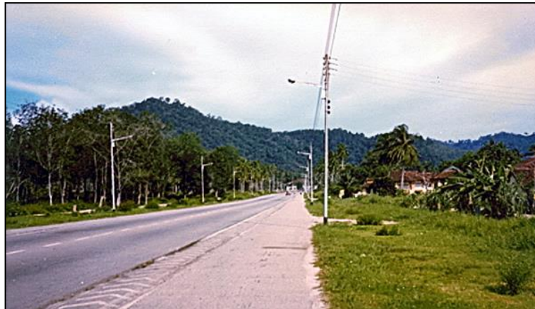
Figure 1.1: Federal Route 50 being two-lane undivided roadway before upgrade ( www.batupahat.org )
