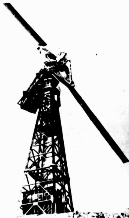
Figure 16. - 1250 kW wind electric generator, Vermont, 1941.
