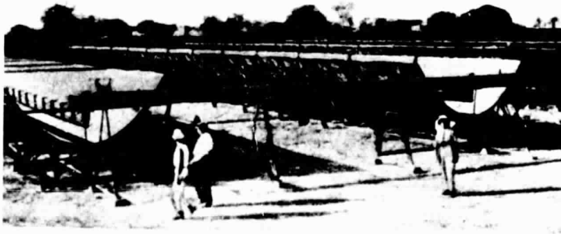
Figure 11. - Focusing solar collector system used to operate 100 hp steam powered irrigation pump, Egypt, 1913.
