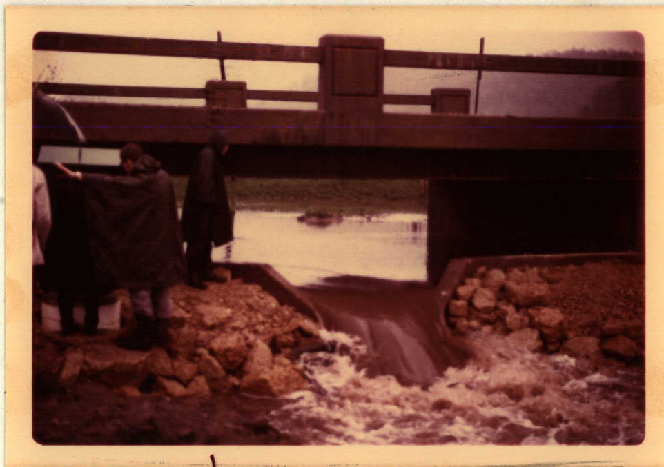
Figure 2. Streamflow gauging station. Type "HL" flume with supporting structures. Site location is shown in Figure 1.
