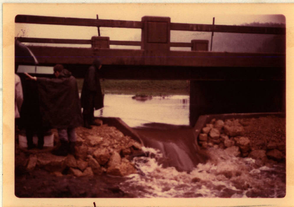
Figure 2. Streamflow gauging station. Type "HL" flume with supporting structures. Site location is shown in Figure 1.
