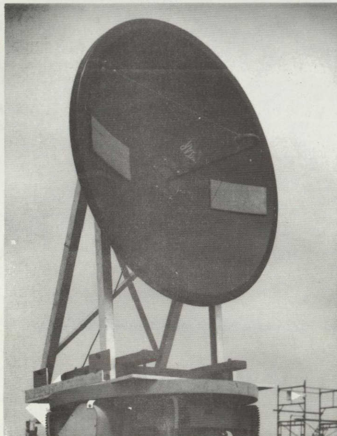
Fig. (3-18)--Reflector with absorbers mounted.
