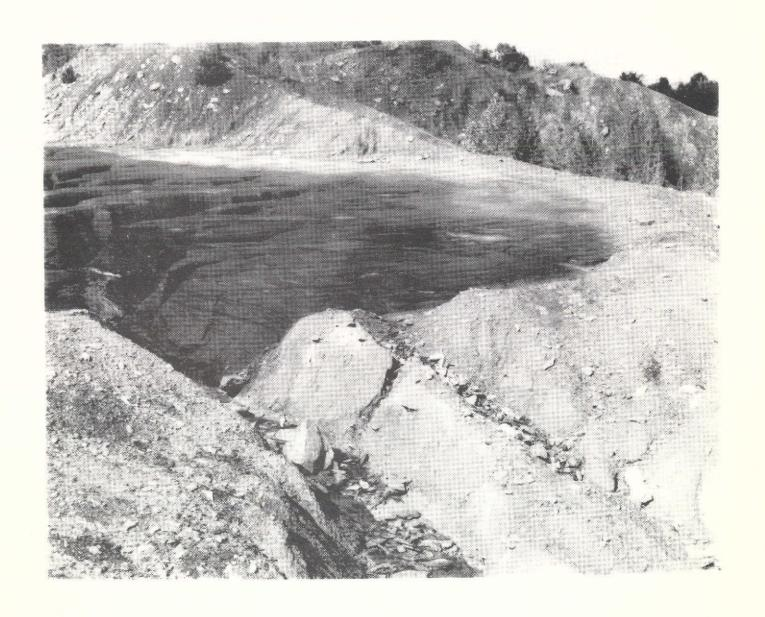
Figure 6.1. This breached slurry containment dam in Kentucky graphically illustrates the type of problem that can develop from old coal preparation sites. Here, thousands of cubic yards of toxic waste material is being eroded into a drainage system.
