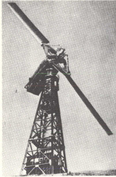
Figure 5. - American Smith-Putnam wind generator 1.25 MW (30 mph wind).
