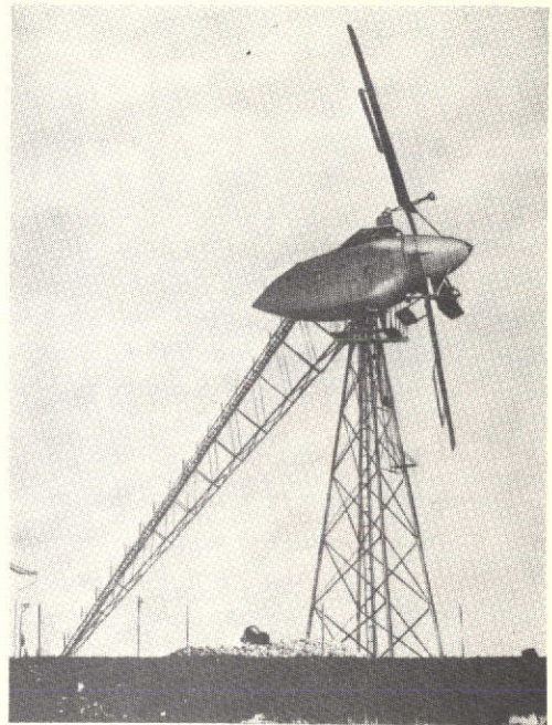
Figure 2. - 100 kW (24.6 mph wind) Russian wind generator.
