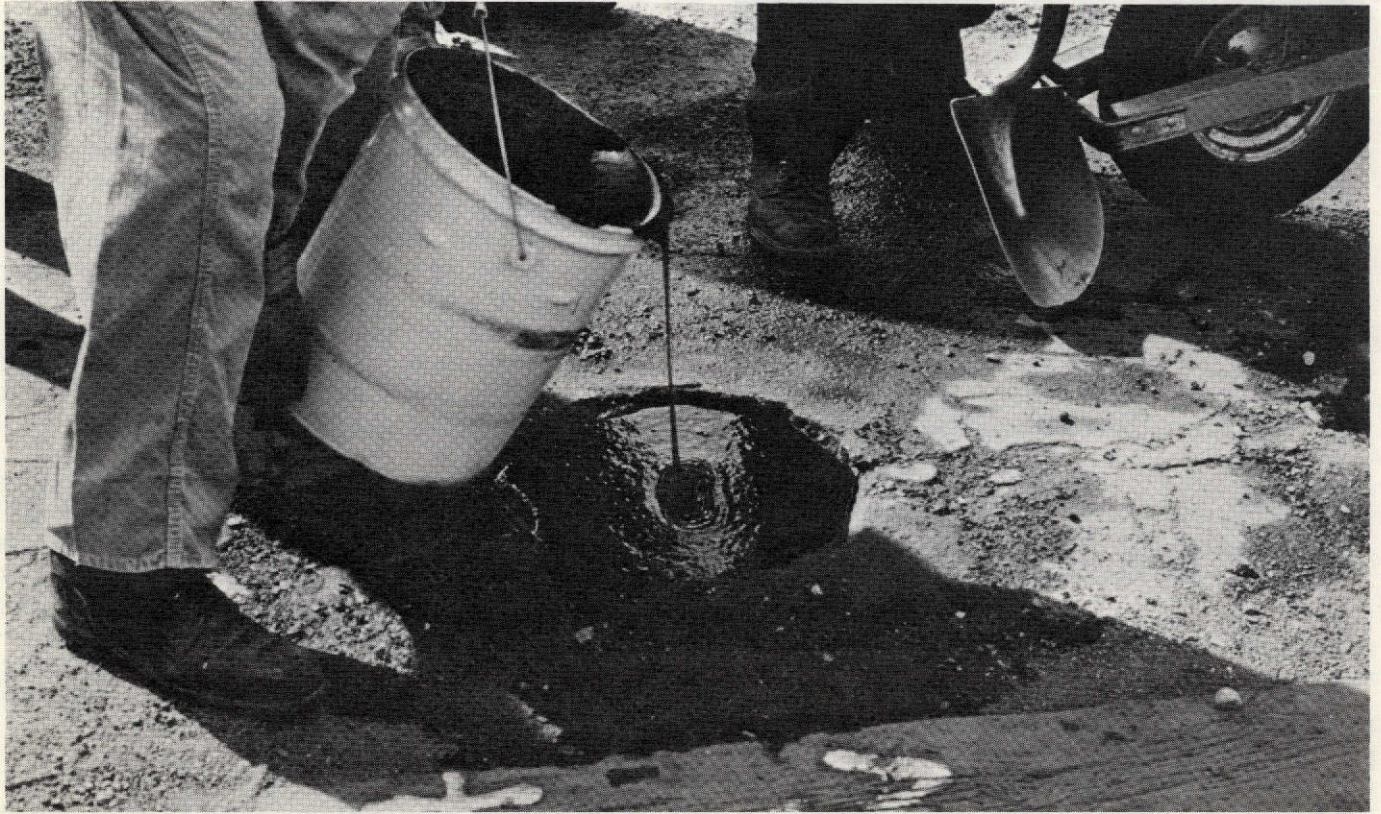
Figure 8. Thermoplastic material originally developed for binding solid fuels for rockets is being adapted for bridge-surface coating and road repair. A potential bonus is that shredded tires and used crankcase oil might be used as an ingredient.
