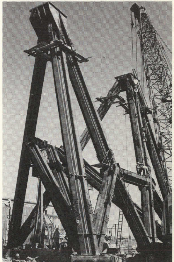
Fig. 19. Alidade during trial erection
