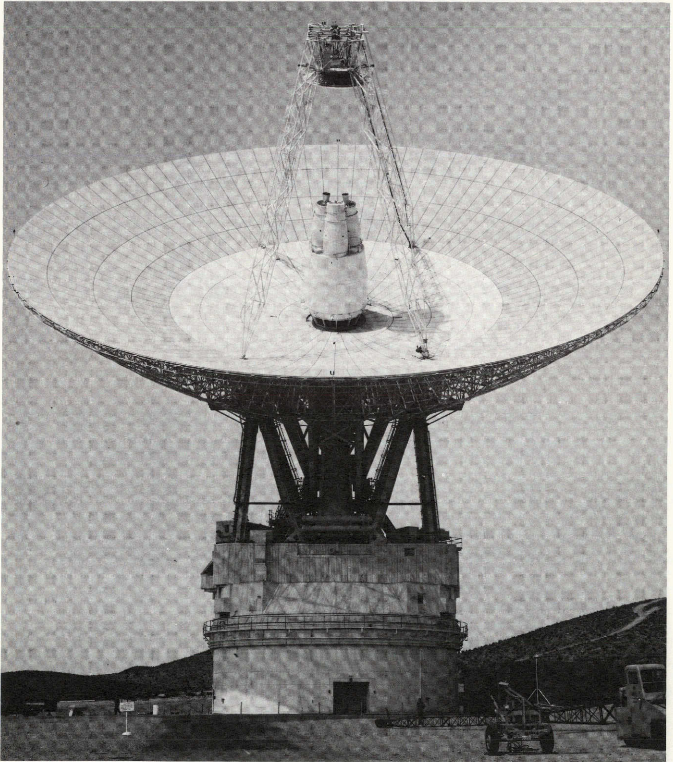
Fig. 158. Tricone installed on the 64-m antenna
