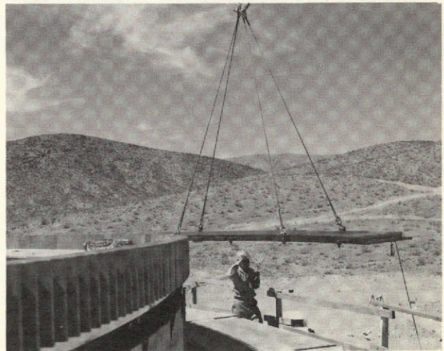
Fig. 25. Hydrostatic bearing runner being placed
