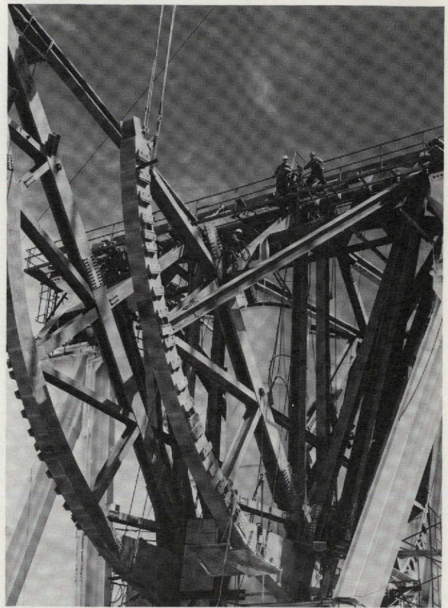
(b) Elevation wheel being installed
