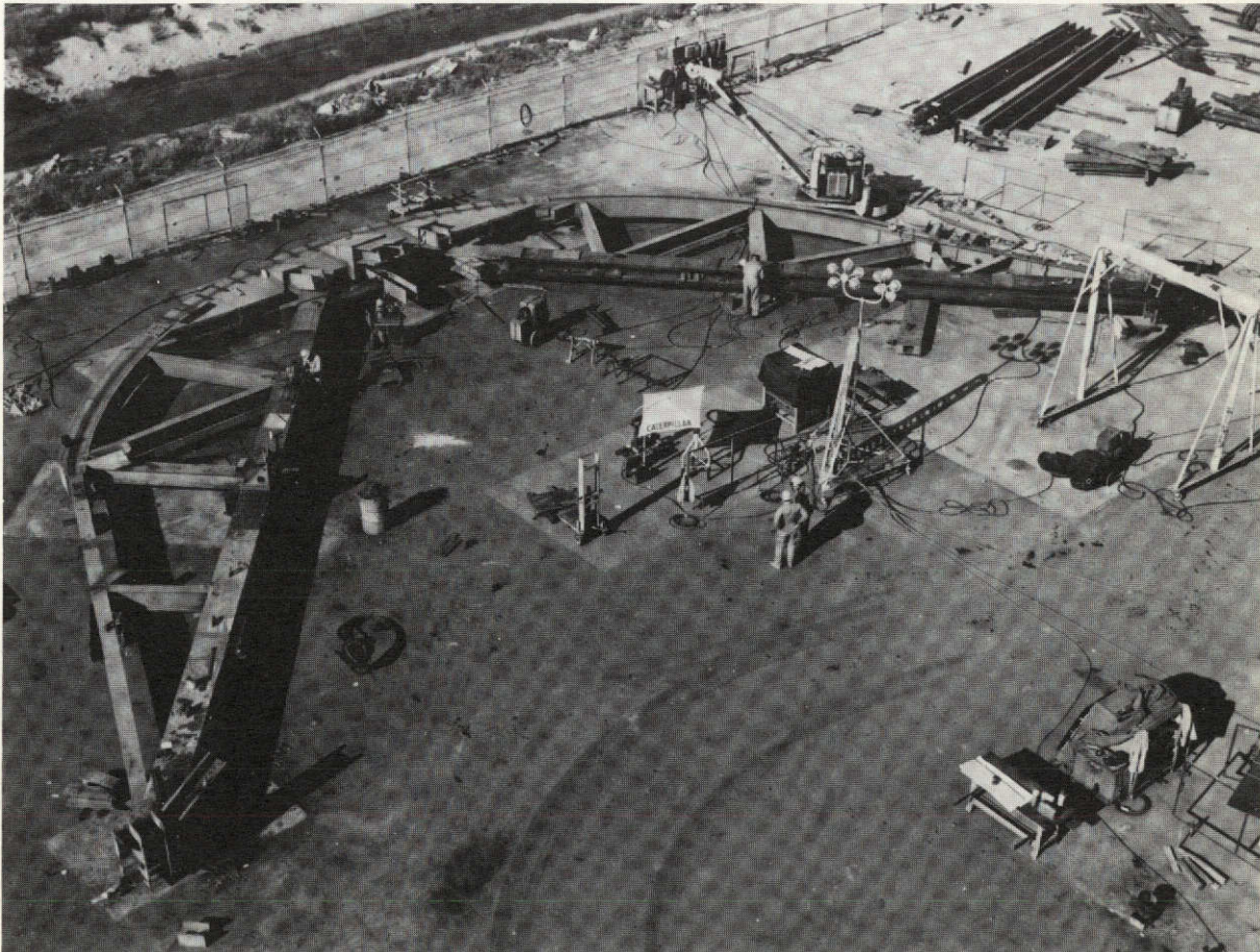
Fig. 42. Elevation wheel being fabricated
