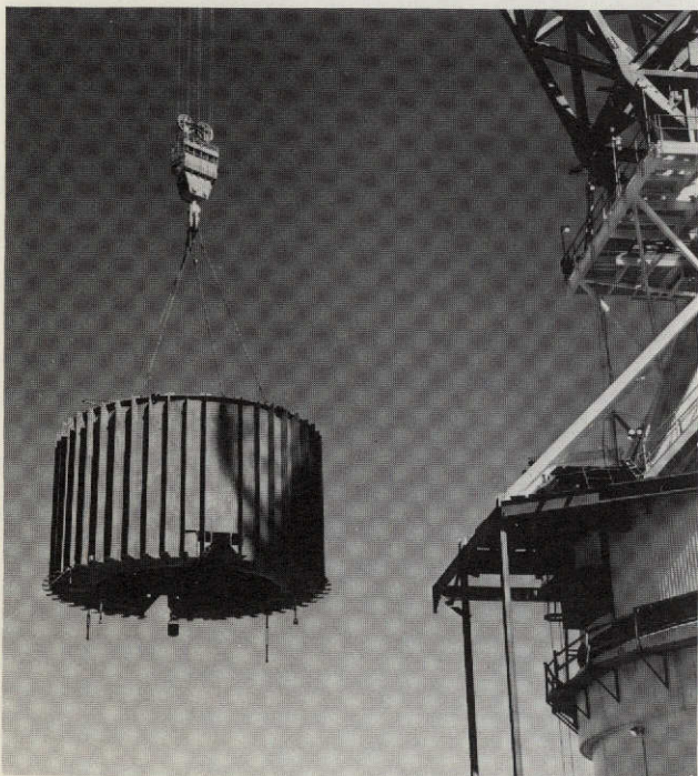
(c) Lifting the center hub
