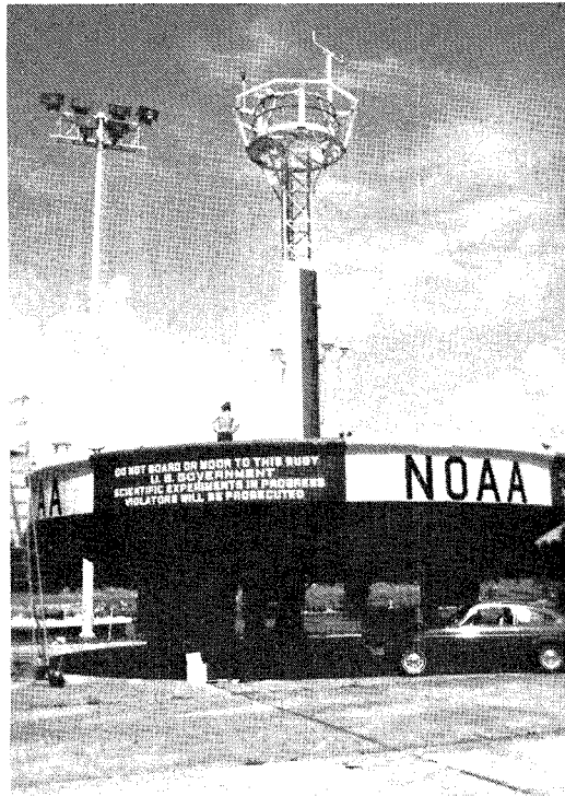
Figure 11(a). - NOAA experimental buoy with solar cell powered simulated RAMOS system.
