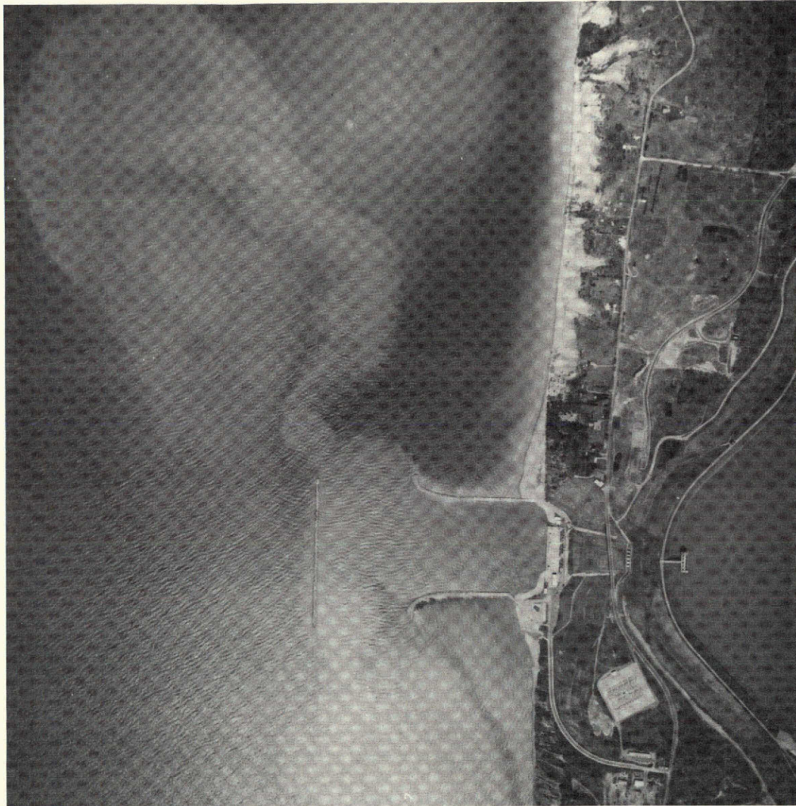
FIGURE 4. LUDINGTON PUMP STORAGE PLANT, 24 APRIL 1974. The Ludington Pump Storage Plant acts as an energy storage system by alternately transferring large amounts of water between Lake Michigan and the elevated reservoir at the right. The large structure and the intake or discharge of water can substantially alter the lake circulation patterns, which are predominantly northward during the summer. Continued monitoring of the effect of the plant on these patterns is important to determine the degree to which they cut off littoral transport of material and contribute to shore erosion in the vicinity of Ludington, a few kilometers to the north. (Original in color.)
