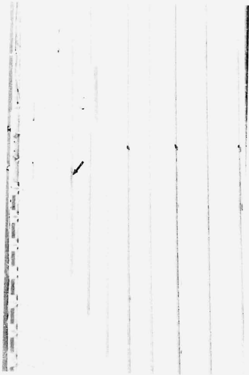
FIGURE 5 LOCATION OF FAILED TUBE 5, PANEL 6
