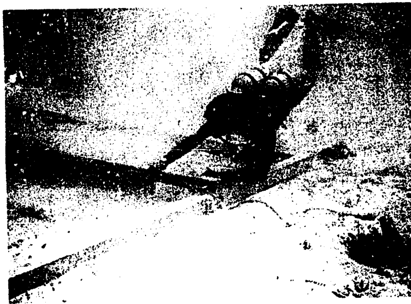
Fig. B53 - Habitat site being leveled by moving a screed bar along a level frame
