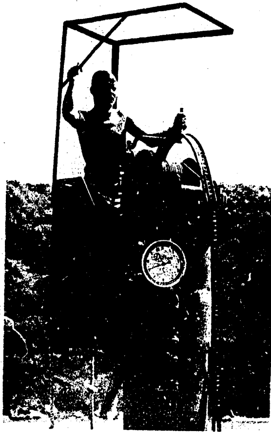
Fig. B51 - Tensionometer in use to control the descent of the launch barge
