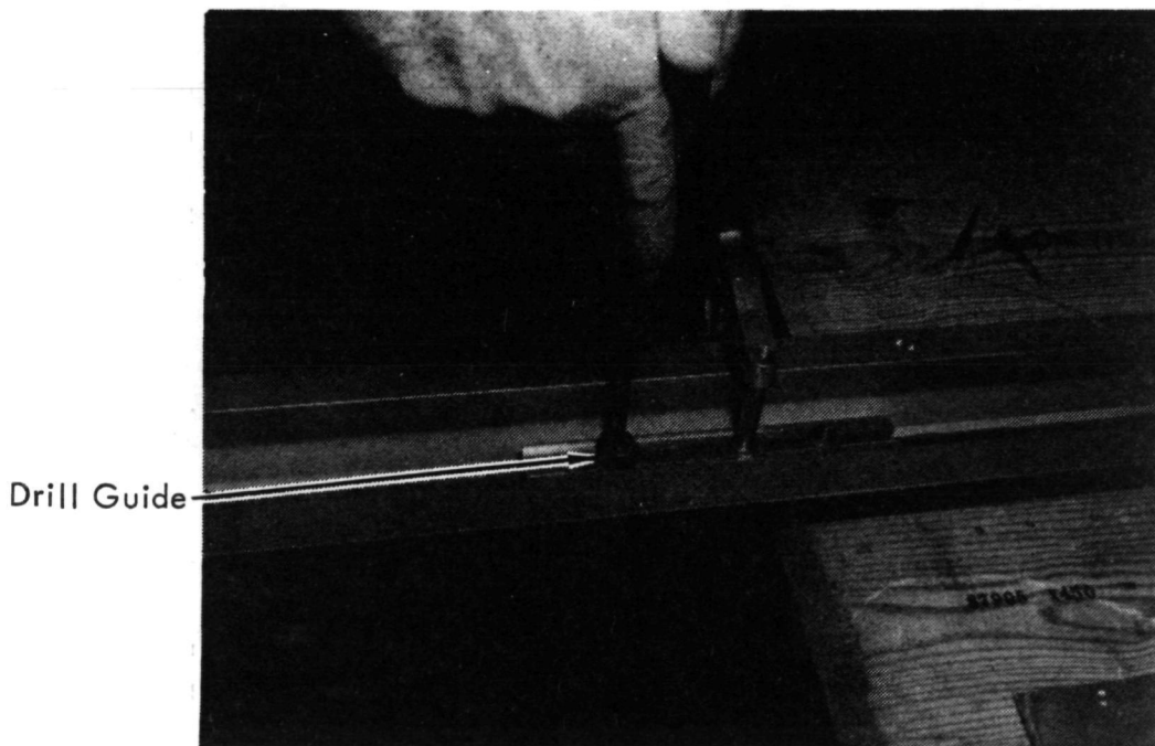
FIGURE 48. - DRILLING HOLES AT LAMINATE END
