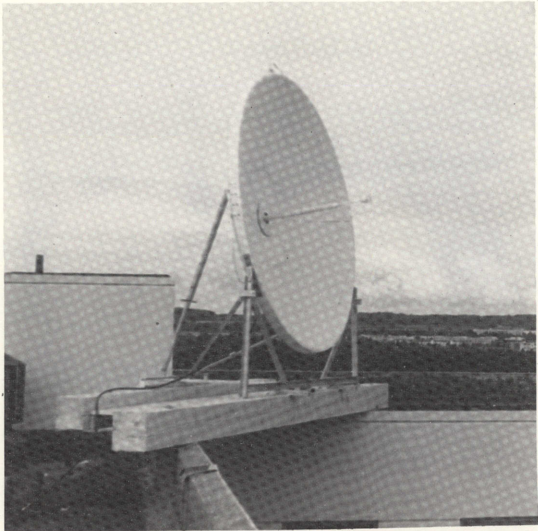
Figure 20-14. S-band Antenna at Anchorage General Hospital
