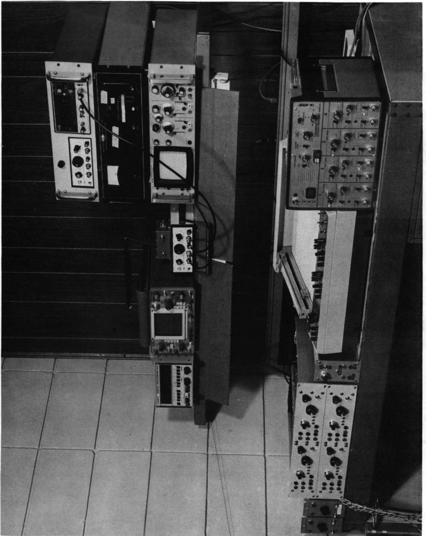
Figure 35 Phase I and Phase II Test Instrumentation
