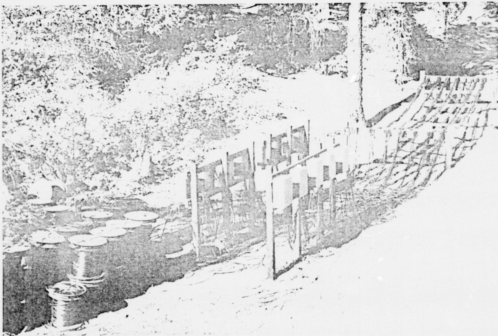
Figure 23. Typical cable installation at TFSO
