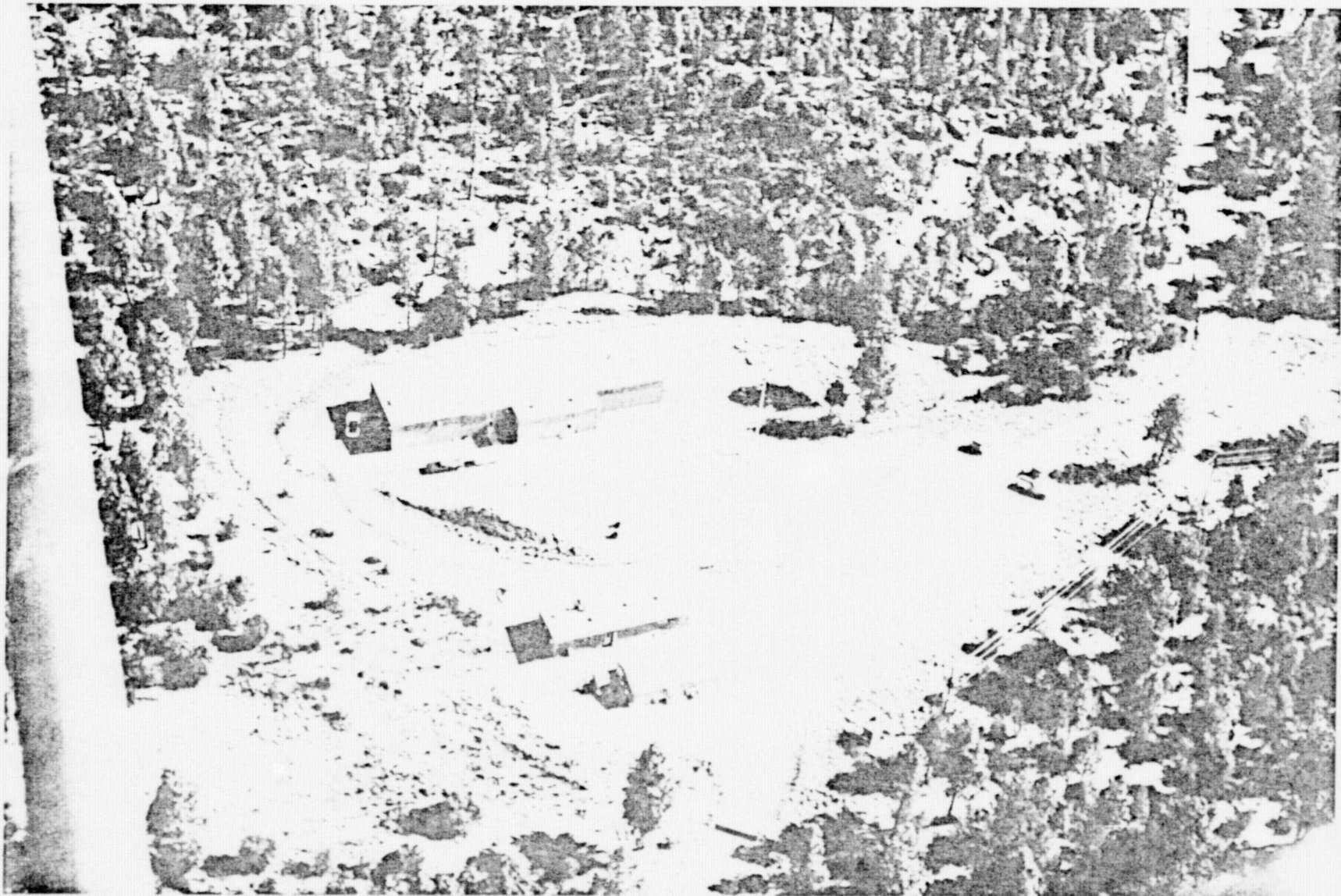
Figure 19. Central facility at TFSO
