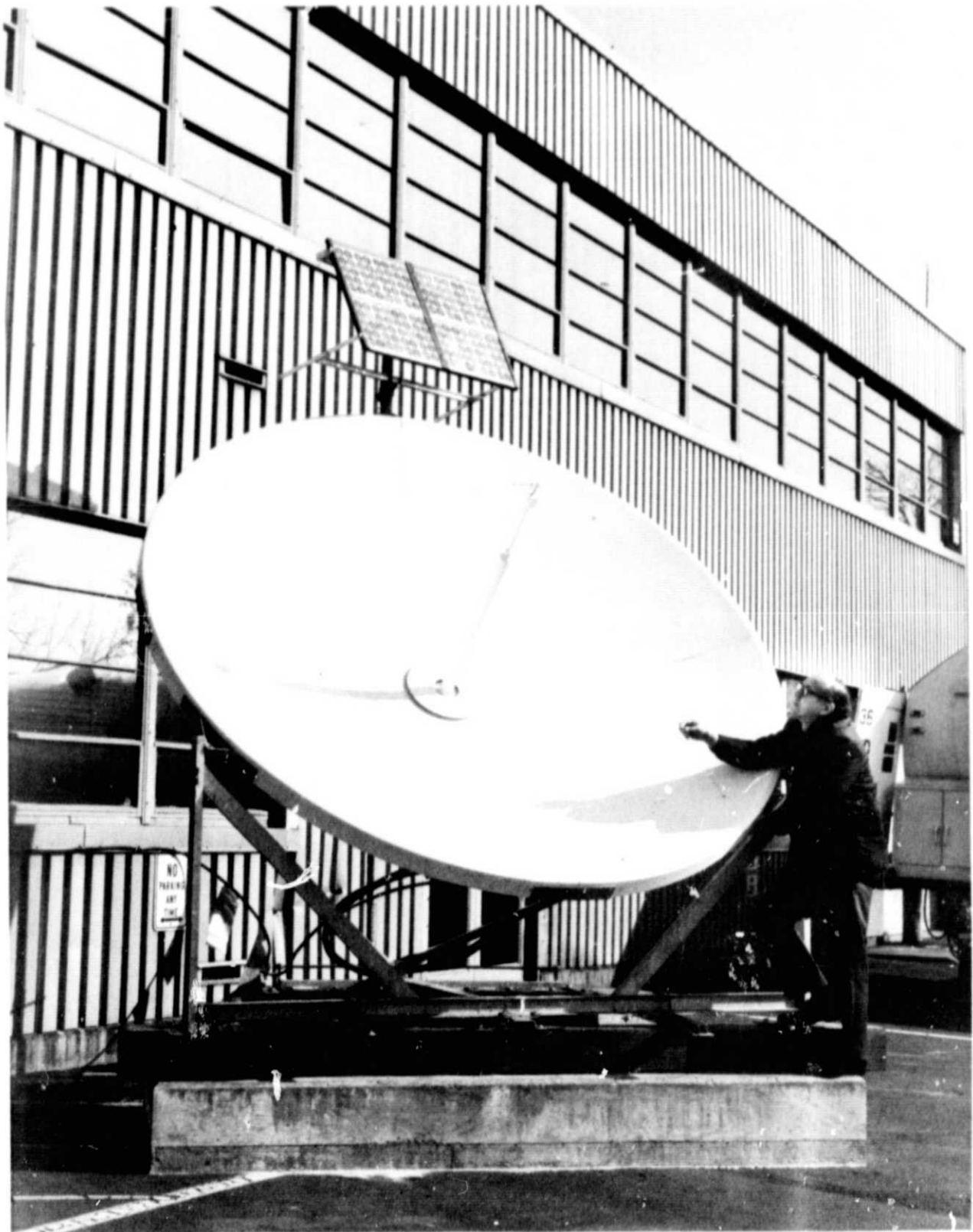
Figure 1. - Demonstration System of HET Receiver Terminal
