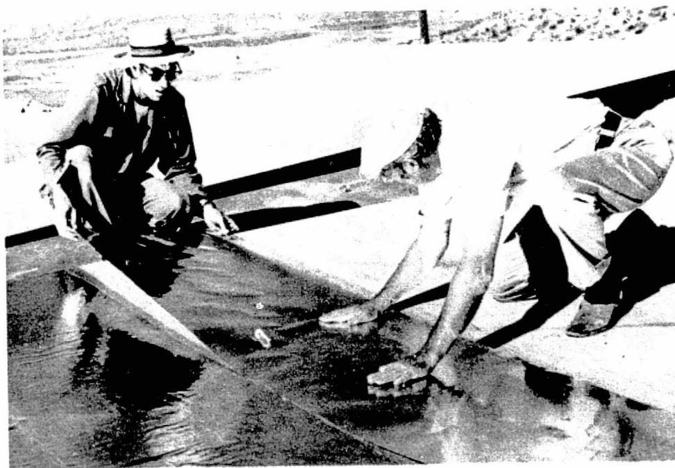
Fig. 2-9 Cementing Aluminum Foil to Bucket Interior Surface (13 Nov. 1974)
