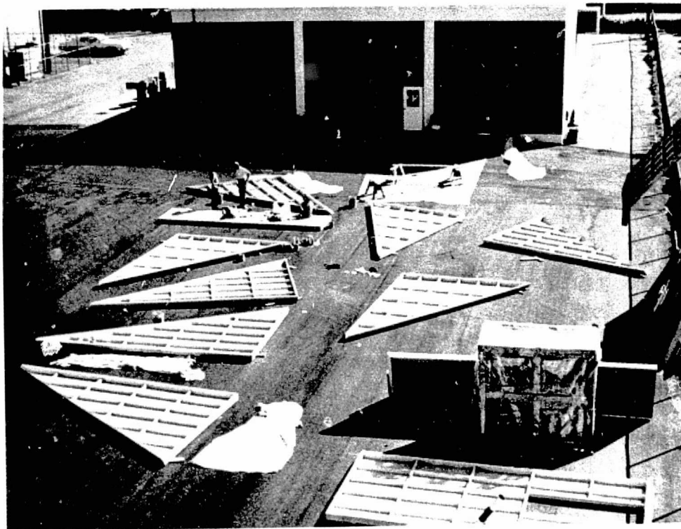
Fig. 2-8 Pre-fabrication and Painting Bucket Parts (12 Nov. 1974)
