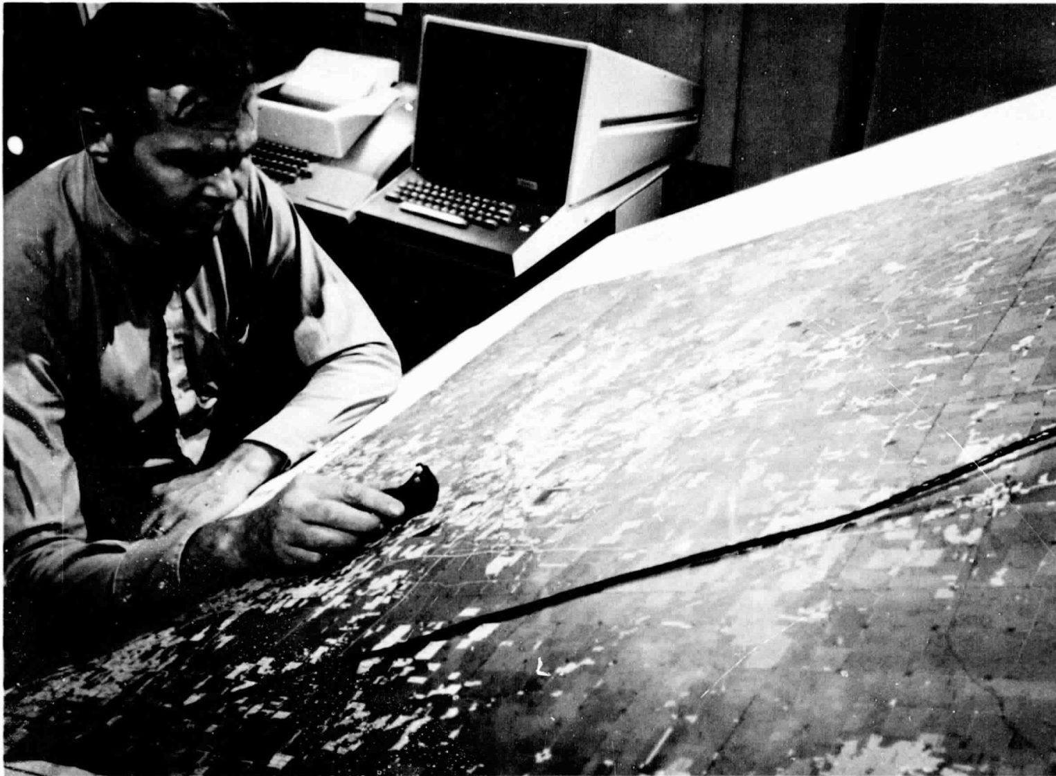
Figure 5-9 Bendix Datagrid Digitizer System Being Used to Digitize Boundaries of Areas for Which Area Printout Tables Are Required
