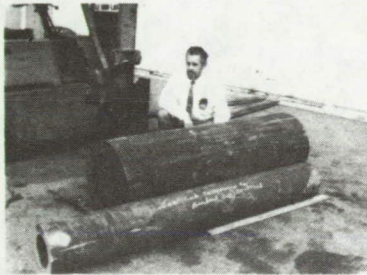
BLADE ROOT END FORGINGS
