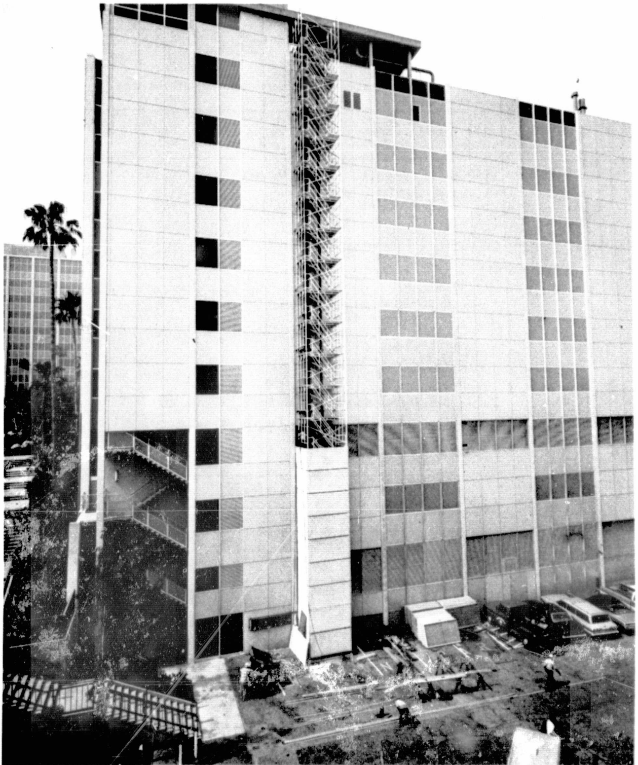
Fig. 1. VICS-120 facility under construction
