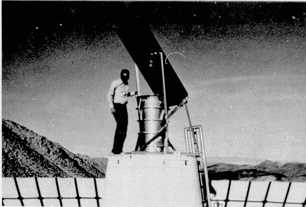
Figure 10. DSS 13 flat plate reflector on SRO feedcone
