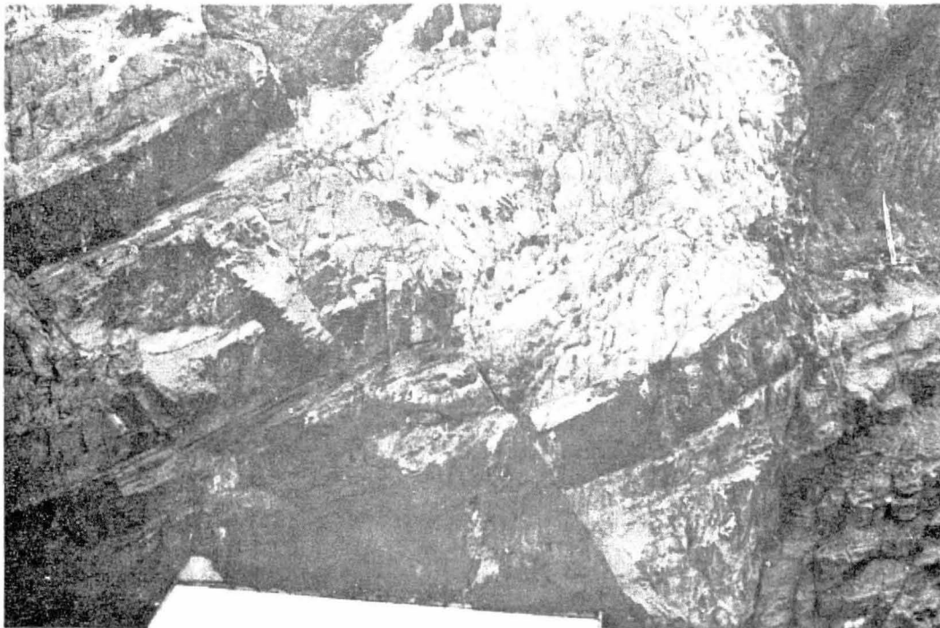
b) FAULTED DIKES ON ARIZONA SIDE OF HOOVER DAM
