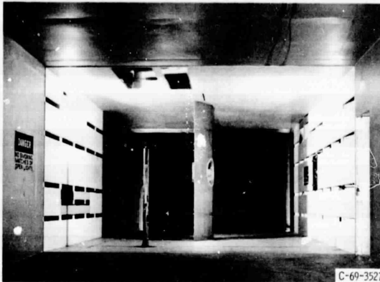
(a) INTERIOR VIEW OF 9x15 FOOT TEST SECTION SHOWING PLYWOOD WALLS.
