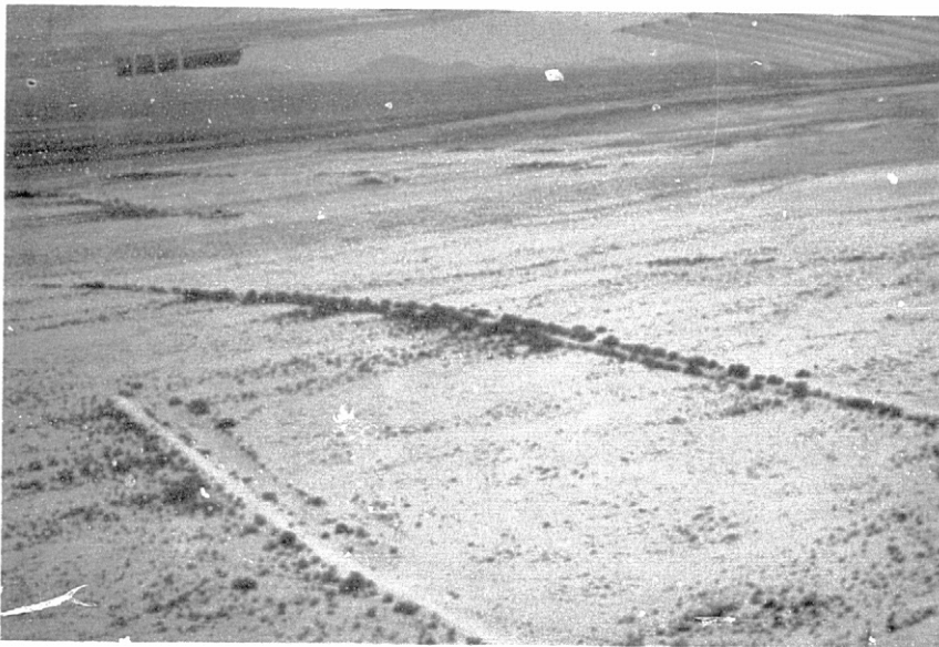
Figure 25. Infrared aerial photo of two downstream diversion structures (#7).
