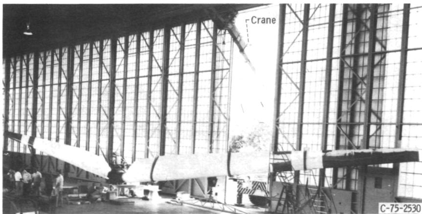
Figure 26. - Blades fitted to hub.
