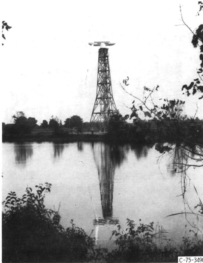
Figure 1. - ERDA-NASA 100-kilowatt experimental wind turbine.
