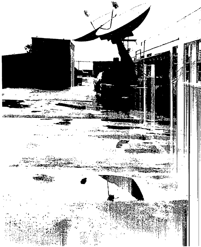
Figure 1a. Balcones Research Center antenna system.
