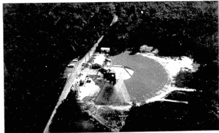
View From West
