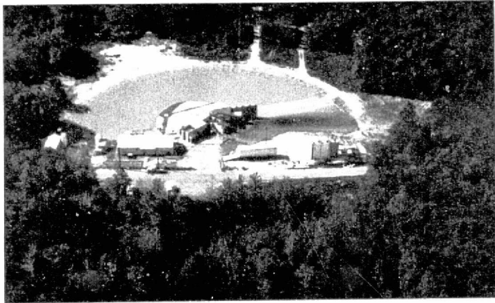
View From North
